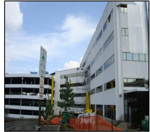
Photo 1. Side A of the fire structure; skywalk and parking garage on the left. (NIOSH photo)
