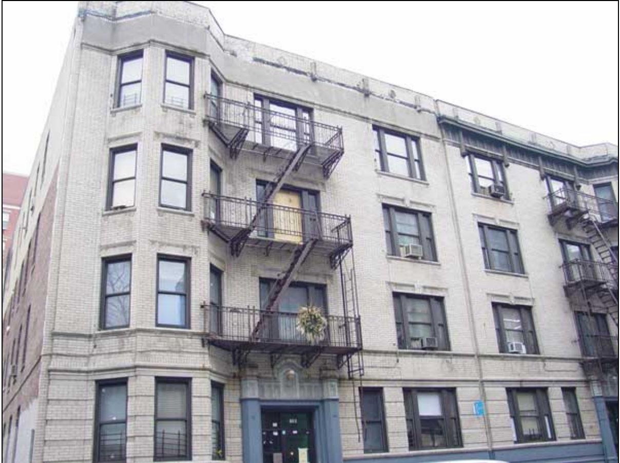
Photo 1. Front of Incident Structure
