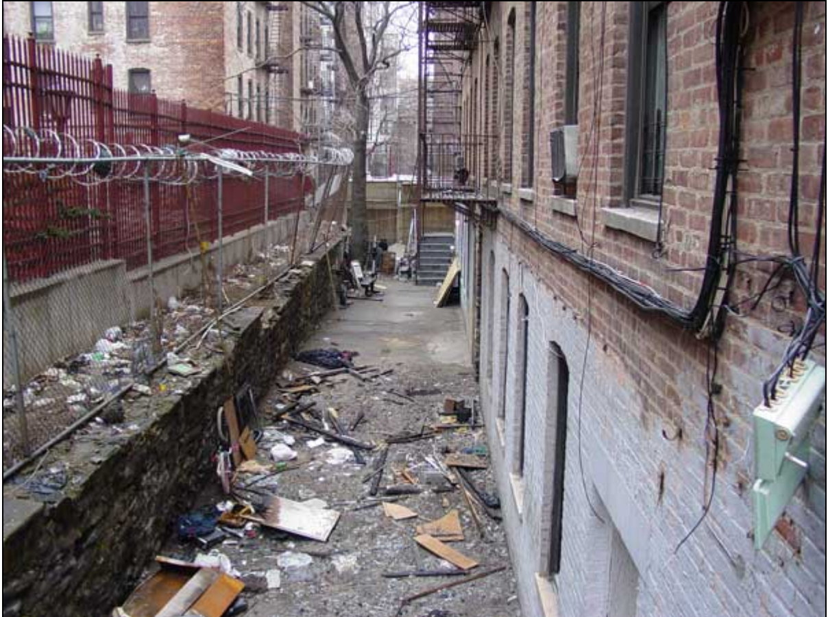
Photo 4. Location in Rear of Structure where Fire Fighters Fell
