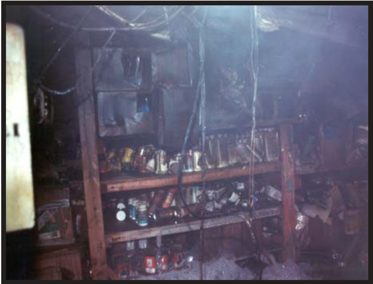
Photo 3. Example of Hazardous/Flammable Materials Stored in Cellar
