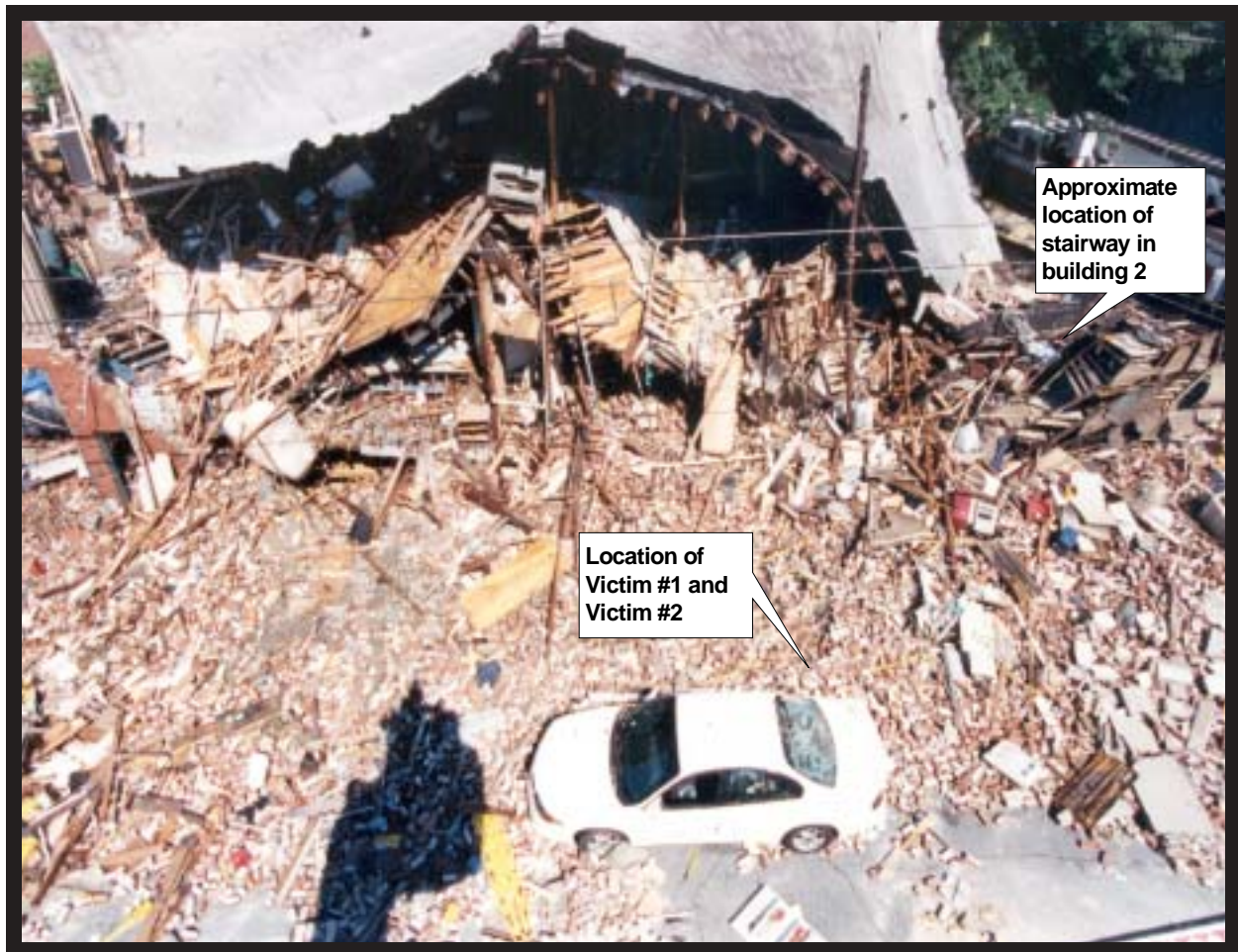
Photo 1. Collapse of Building from Side 2
